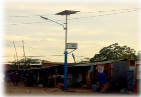
Installation in Rwanda
